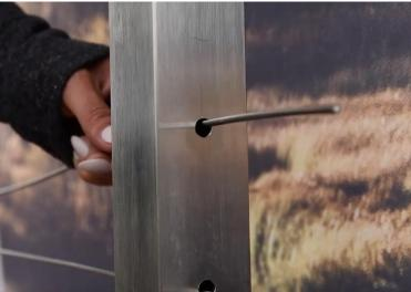
**Step 4. Measure and cut**. Pull the wire rope tight and place a mark approximately where the wire rope meets the post. Make your cut.
