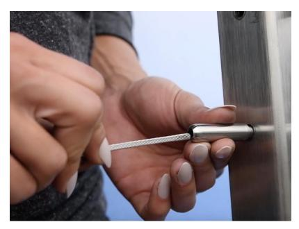
**Step 6- Tension your wires**. Go back to the first post. Starting in the middle and working your way out, grab the wire rope in front of the receiver with a pair of vice grips to hold it still. Using a 10mm wrench, turn the Swivel receiver clockwise until your desired tension is reached. Be careful not to let the wire rope turn as you do this.
