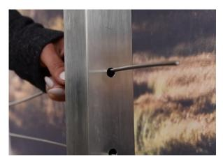
**Step 4. Measure and cut**. Pull the wire rope tight and place a mark approximately 1.5" past the start of the Self-grip receiver. Make your cut.
