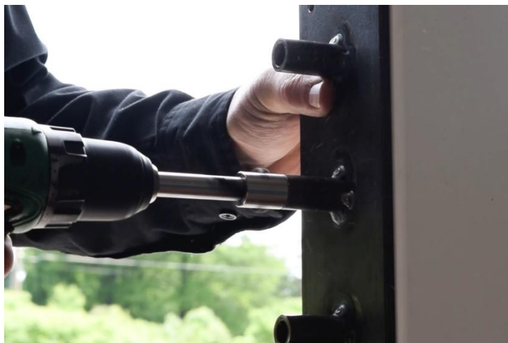
Photo shows drilling counter holes using our drill template and our drill stop.
