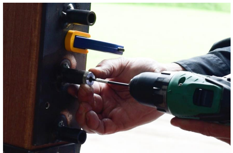
This photo shows the pilot holes being drilled using our drill guide.
