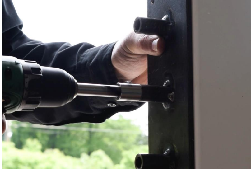
Photo demonstrating using our drill template and drill stop to make counter holes
