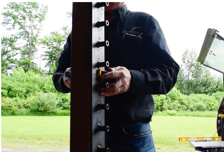
This photo shows the pilot holes being drilled using our drill guide.
