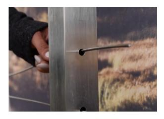
**Step 4. Measure and cut**. Pull the wire rope tight and place a mark approximately 1.5" past the start of the swivel receiver. Make your cut.
