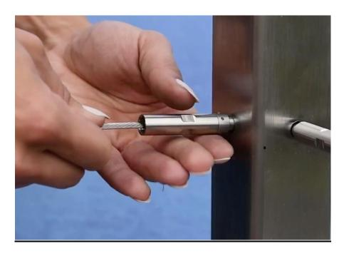
**Step 6- Tension your wires**. Go back to the first post. Starting in the middle and working your way out, grab the wire rope in front of the receiver with a pair of vice grips to hold it still. Using a 10mm wrench, turn the Swivel receiver clockwise until your desired tension is reached. Be careful not to let the wire rope turn as you do this.
